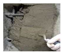
Sika produces an extensive range of prebatched hand trowel applied repair systems for localised patch repairs. These include chemically resistant materials to protect against aggressive acidic gases and liquids. The most frequently used systems for these structures are **Sika MonoTop**® cementitious mortars for general repairs and **Sikadur**® epoxy resin based mortars for chemically exposed repairs.
