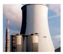
Zone 2 – The middle section, normally 5 – 30 m and Zone 3 – the rest of the external surfaces, up to 70% of the surface area. The ideal combination of **Sikagard®** hydrophobic impregnations followed by **Sikagard®-680 S** is widely used for the bulk of the external surfaces and this also conforms to the OS2 classification of the German Federal Regulations for concrete protective coating systems. **Sikagard®-550 W** elastic coating is used where additional crack bridging performance is required.
