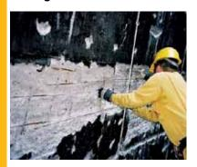
Complete surface cleaning and damage area identification and marking for removal or further investigation. Following the results of the Engineer's Condition Survey all of the damaged concrete must be removed following structural guidelines and any exposed steel reinforcement cleaned thoroughly – preferably by blastcleaning to a standard equivalent to SA 2¹/2. (In accordance with EN ISO 8501-1).
